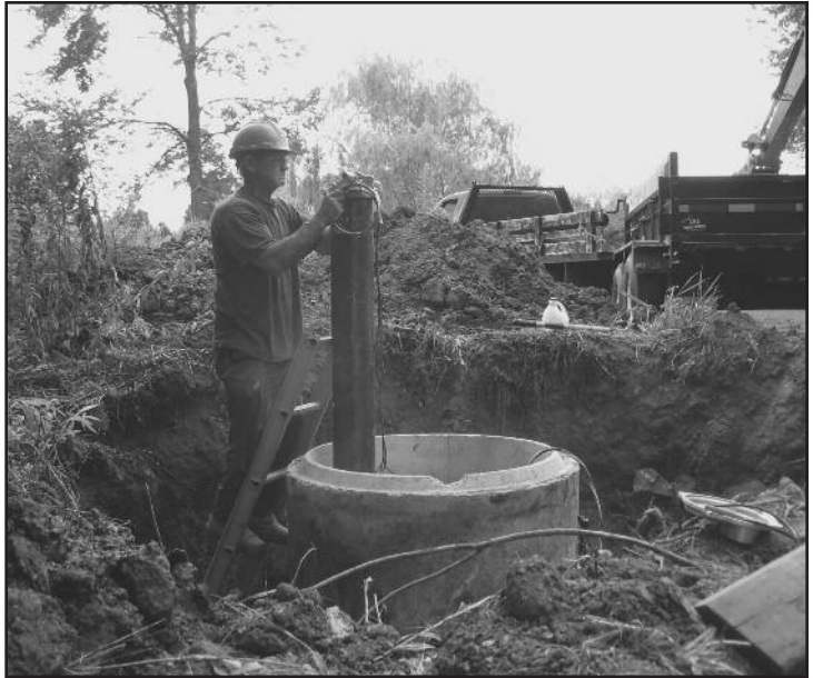
Well upgrade in progress.
