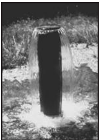
Flowing well that is not controlled.
