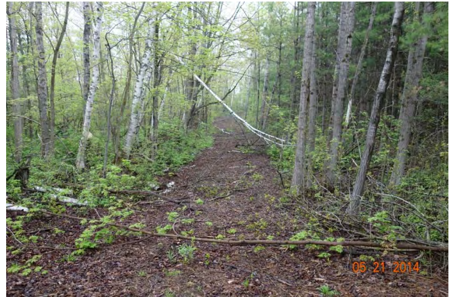
Photo 18 – View of buried feeder line leading to Recharge Well RW206C. This photo was taken 5 years after the feeder line was installed. Note the woody debris and native ground flora along the feeder line alignment. GHD 2014-05-21
