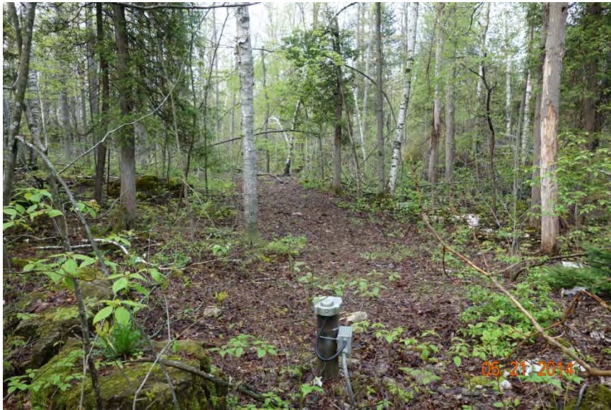
Photo 33 – View of Recharge Well RW207C, taken 5 years after installation in 2009. Note the regeneration of Alternate-leaved Dogwood, Bracken and sedges. GHD 2014-05-21
