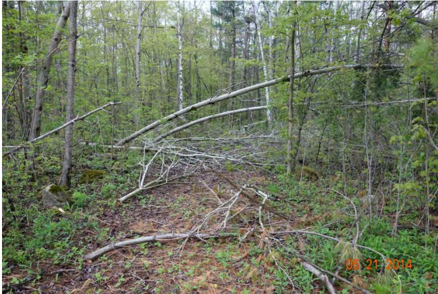
Photo 31 – View of Recharge Well 201C, 5 years after installation in 2009. Note the woody debris and regeneration of forest plants. GHD 2014-05-21
