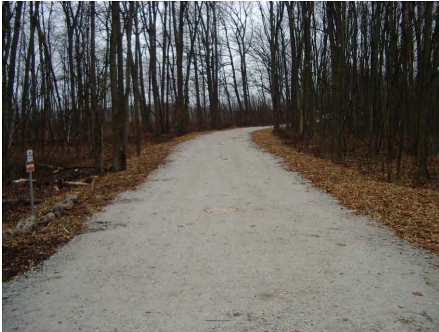
Photo 1 – A view of the East Cell driving access and watermain near Wetland V2, immediately after construction in late 2010. Disturbance is generally contained within a 10 m wide zone, but in this area it was restricted to less than 8 m because it is not adjacent to the extraction area and the alignment was through a treed area. The driving access is generally between 4.0 and 4.5 m wide. The shoulders were treated with 15+ cm of fresh wood chips to curtail the spread of invasive plant species such as Garlic Mustard ( Alliaria petiolata ).
