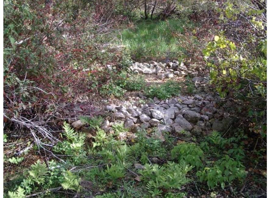
Photo 24 – View of Wetland W7 Diffuse Discharge Inflow, approximately 4 years after it was installed. Note the patch of Sensitive Fern and other wetland plants that have colonized the feeder line alignment. GEC 2014-09-22
