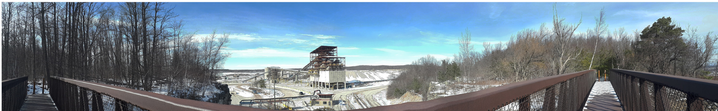
Photo 15: Taken on Dufferin Bridge facing towards existing quarry and future extension.
